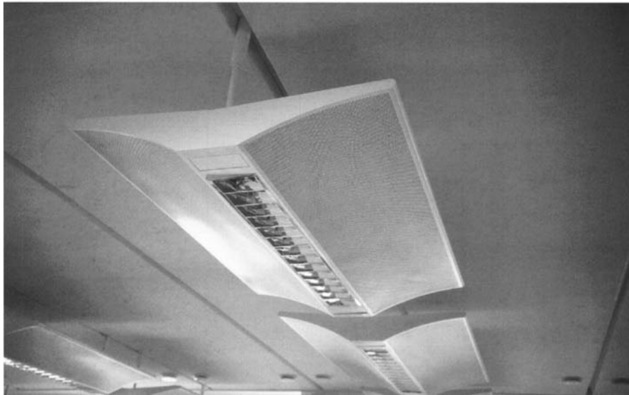
9: Close-up of luminaire with acoustic 'wings'
