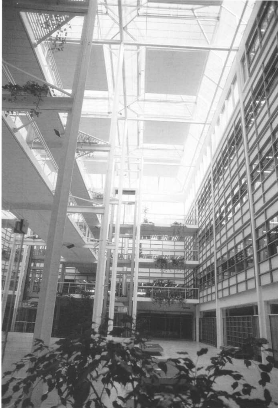
9.20 Gateway 2 at Basingstoke where stack effect in the atrium draws air through the adjacent offices (Architects:Arup Associates).
