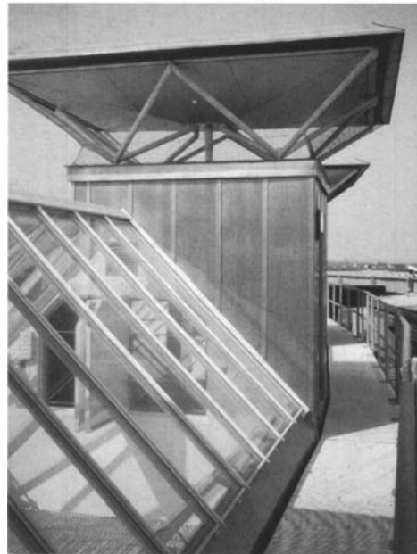
7.12 The Ionica building in Cambridge uses large ventilator elements located on the roof to ventilate internal spaces via an atrium acting as an extract plenum or chimney.
