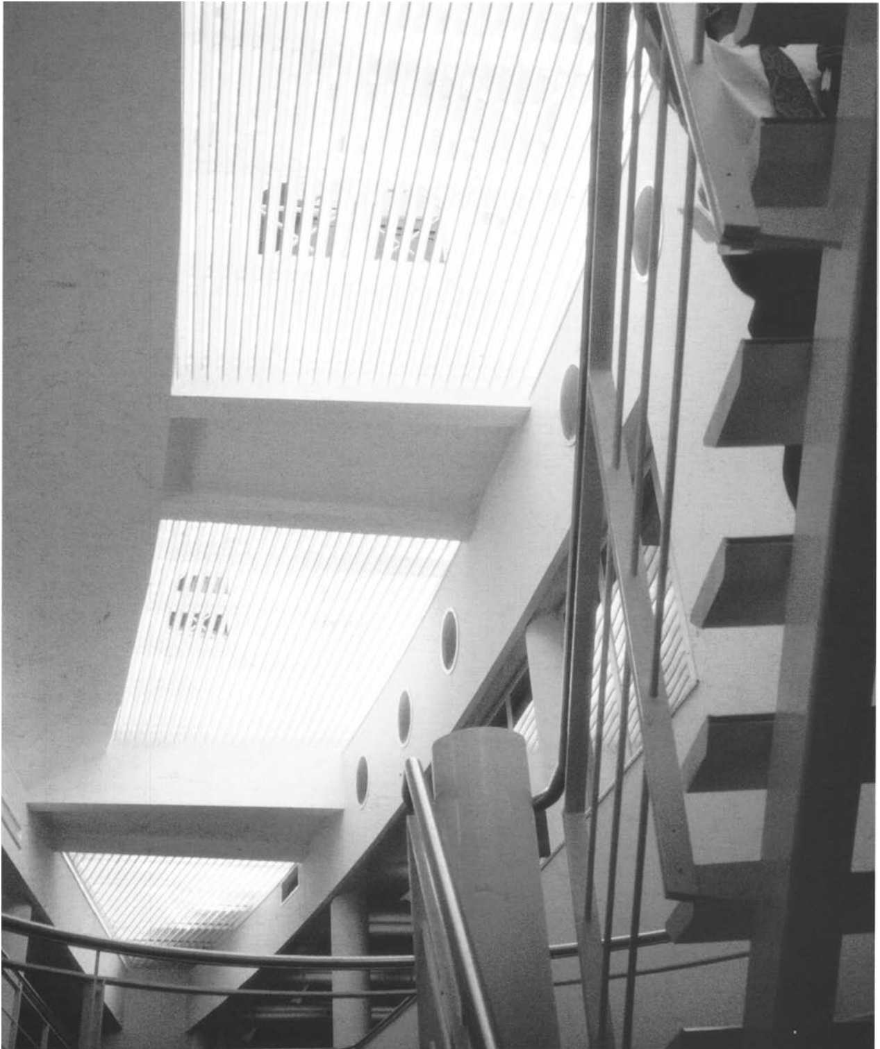
7: Detailed interior view of atrium shading
